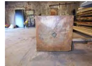
▲ **New Wind Shaft**—The existing wind shaft has been repaired/patched at critical areas in the past. Knowing that at some point it would need to be replaced, we purchased the timber and had it tapered and bored to be ready when it was needed and that time is now.
