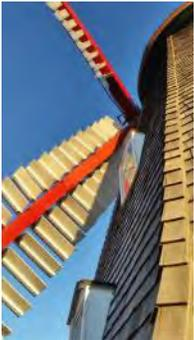
The two 67 foot long timbers of the Danish Windmill sail cross arms weigh 3,500 pounds each and are 80 feet in the air. Wood rot in the timbers posed a major safety concern and jeopardized the integrity of the structure especially in the event of heavy snow.
